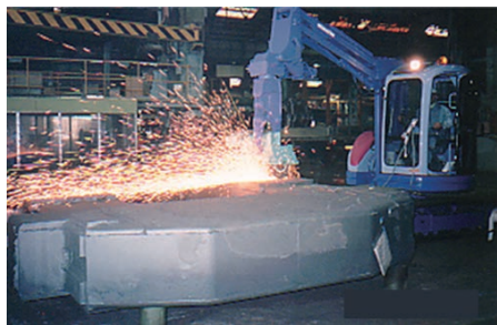
Fig. 13 Grinding work in large machine factory
