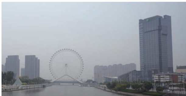
図1 天津Holiday Inn Tianjin Riversideの外観
